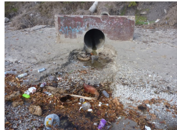
Ropes Park stormwater outfall
