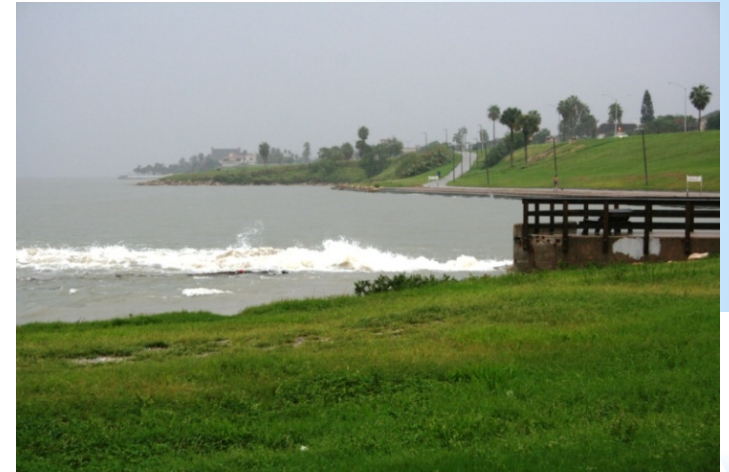
Cole Park stormwater outfall
